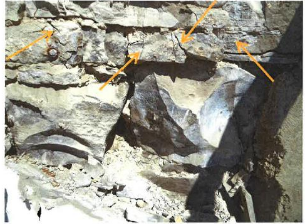
9 Close-up view showing numerous fractures in stone units and poor mortar condition
