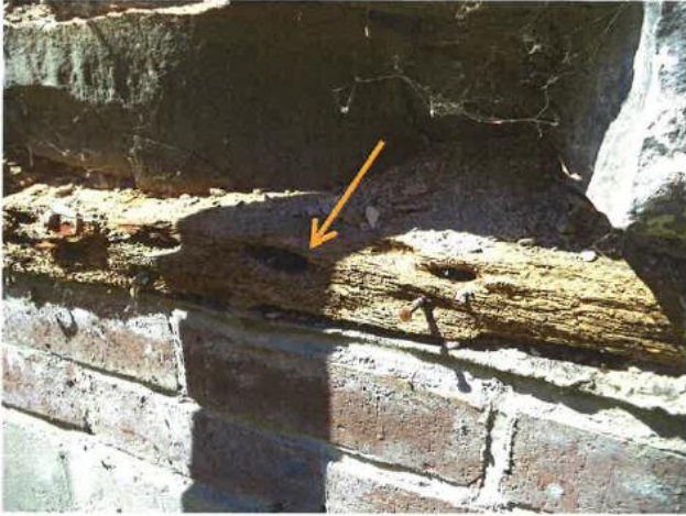
5 Close-up view of decayed wood lintel
